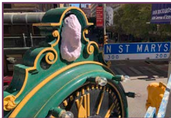
Making a mold of the Hertzberg's Jenny Lind topper
